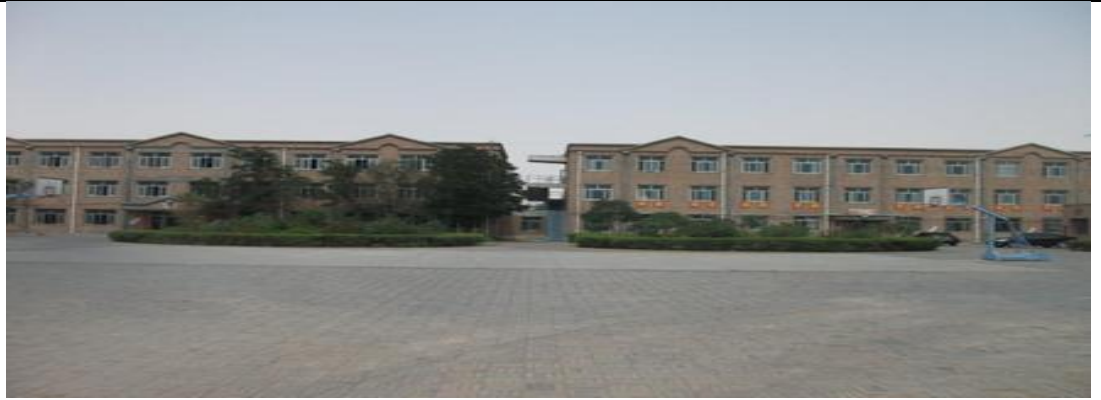
Offices and employee accommodation
